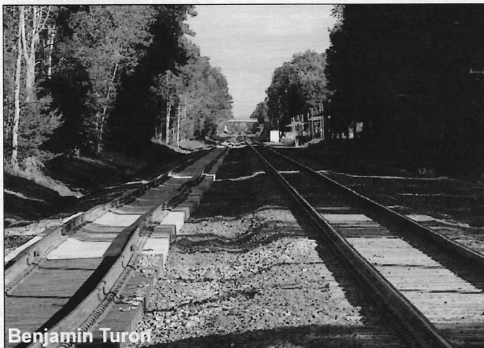
Looking east from Morris Road crossing toward New Karner Road overpass shows new 2nd track to left of existing
