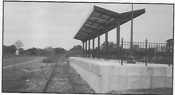
Platform at stadium awaits Park Street Bridge completion
