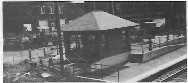
Whitehall Station under construction. Photo Dr. Margarethe McCurry
