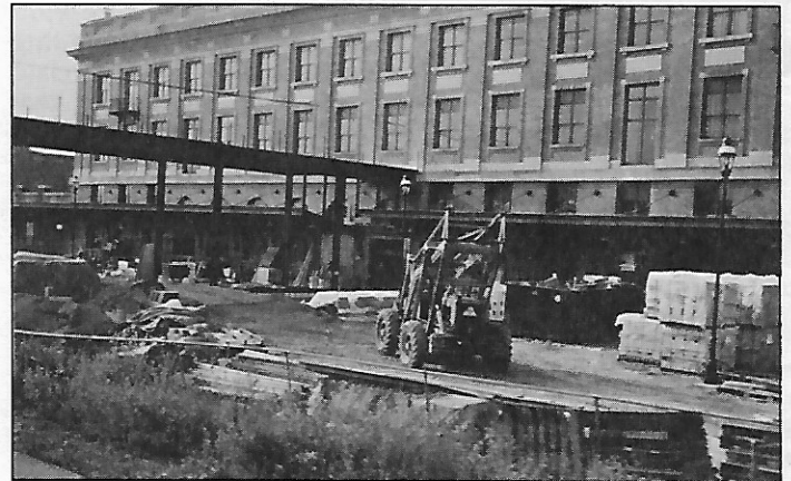
Work continues on the Utica, N.Y. station.
